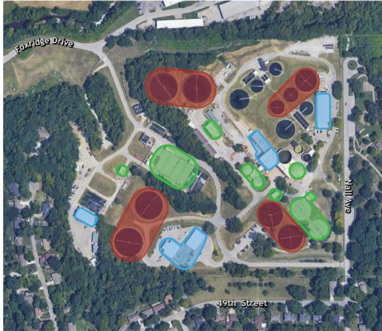
Pre-Construction Nelson Facility
